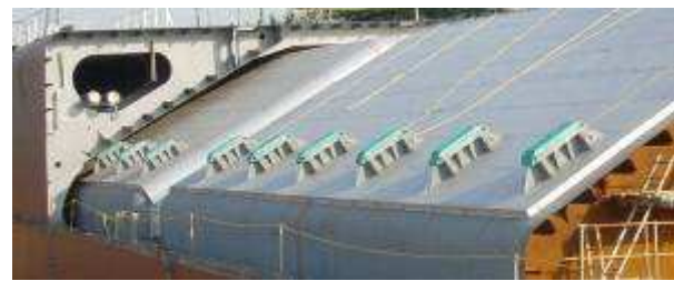
Figure 8: Specific instructions on where to look, what to look for and how to report damages in the tank – 3D graphics and the real vessel
